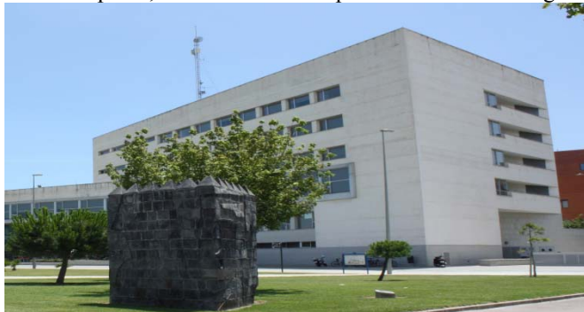
Figure 1 Site location of the transmitter on the top of the building inside of the main campus.
